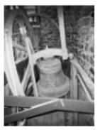
On investigation we found that the treble had dropped from its bearings on one side, with the wheel leaning against the frame and the bell pitched on its slider but resting on the running board where it had dropped down into the frame.
